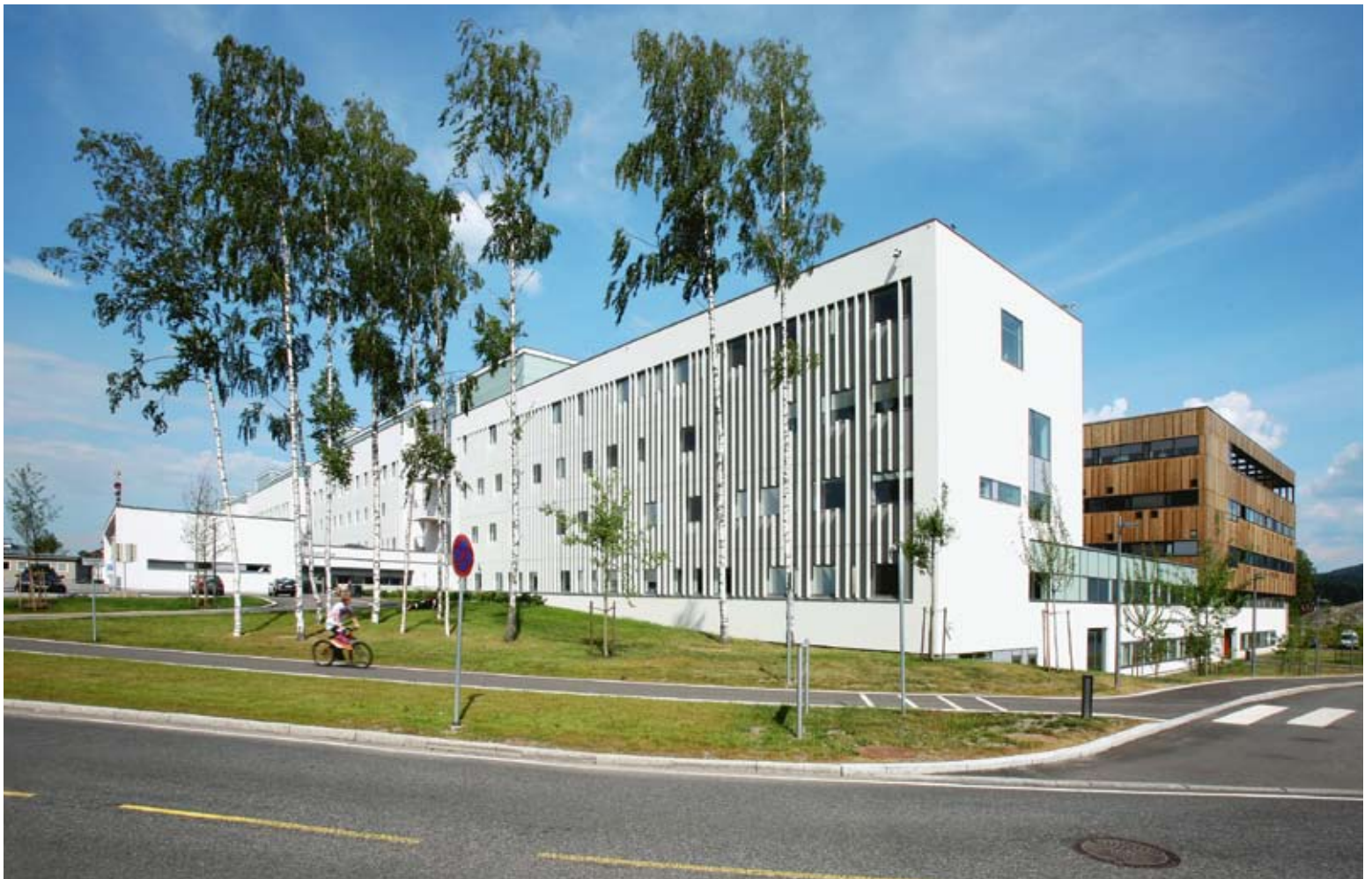
On the west façade, all the windows in a section are gathered into one field, framed by a white plaster area, which is faced with dark grey cement composite panels and shaded by vertical aluminium lath mounted in front.
