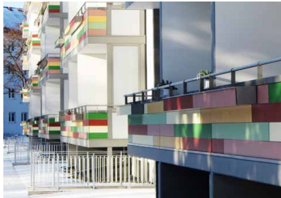
Housing complex | Dresden | Germany
